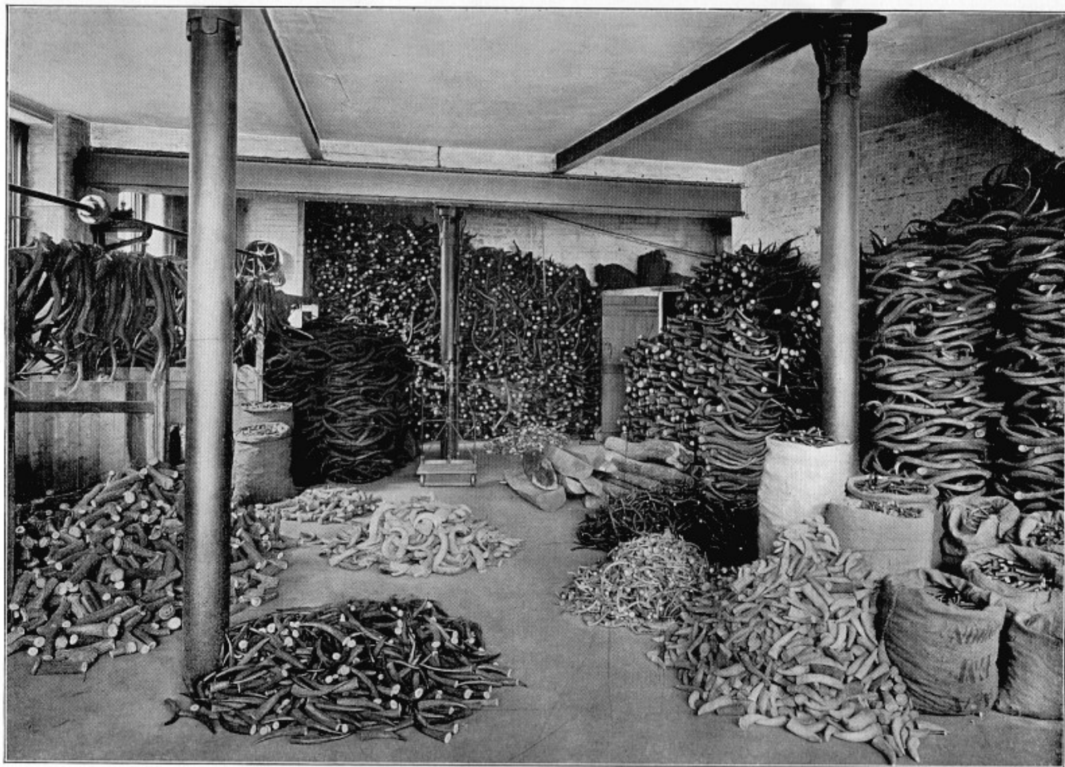
STAG STORE CELLAR, POND HILL WORKS.
